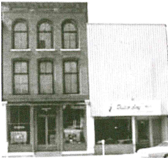
Whereas the façade on the right has been obscured by an aluminum covering, the façade on the left retains desirable elements including cornices and windows.
