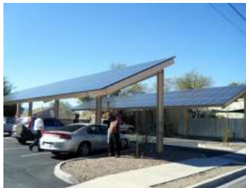
An example of solar panels installed over a parking area
